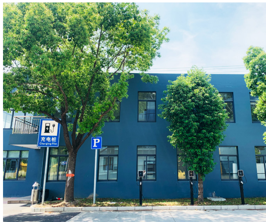
Install Electric Vehicle (EV) Charging Piles in the Factory
